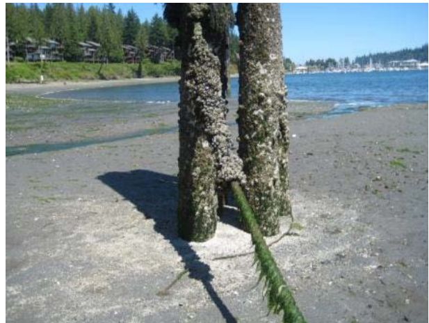
4. Piling #38 Near Creek Minus 2ft-Tide Most-Life
