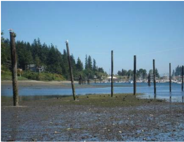
1. Pilings #29-35 Minus 2ft-Tide No-Pile-Life 2 Birds
