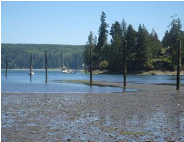
3. Pilings #11-17 Minus 2ft-Tide Little-Pile-Life
