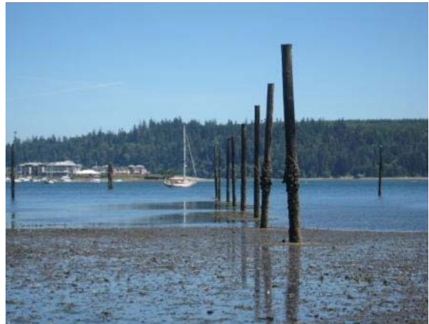
2. Pilings #18-25 Minus 2ft-Tide Little-Pile-Life
